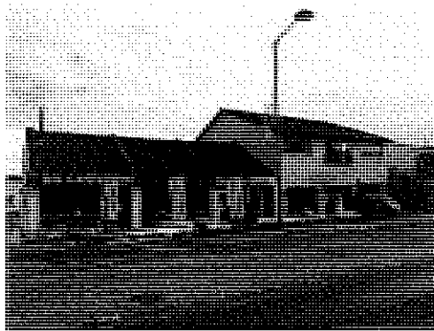
14 Gramplan Road looking south towards retail units.
